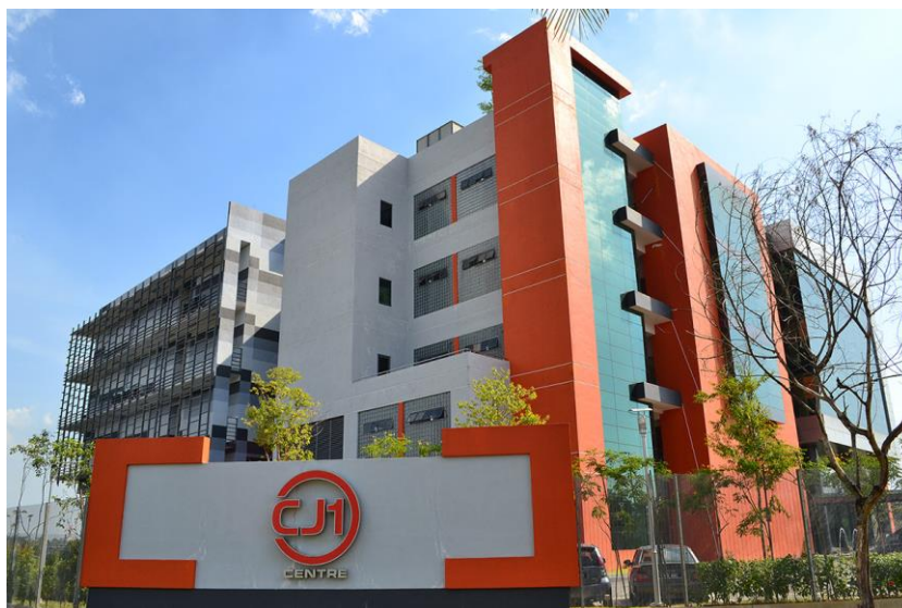
The data center in Cyberjaya
